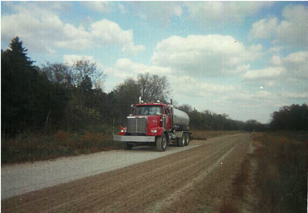
Figure 3. Application of EK ® 35.
