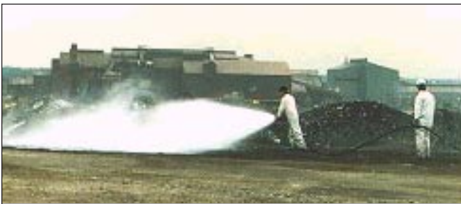
Figure 2. Applying SOIL-SEMENT® to a soil pile.
